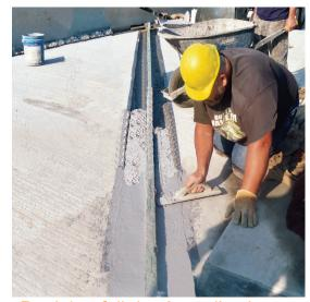
Partial or full depth applications can be accomplished in a single pour restoring the integrity of deteriorated PCC structures.
