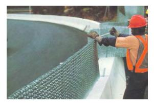
2. Insert <sup>3</sup>/<sub>4</sub>" Post Bolt through the first row of DRC Fabric and attach the End Treatment Cable Anchor Assembly to the top of the <sup>3</sup>/<sub>4</sub> Post Bolt as shown in the detail drawing. Insert the threaded end of the post bolt into the second anchor location. Secure Cable Assembly using <sup>3</sup>/<sub>4</sub>" eye bolt attached to the first expansion anchor in concrete barrier.
