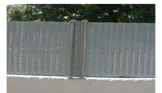
7. When joining two rolls of DRC Fabric, use the splice plates provided (See drawing for anchor locations at splices). Insert the <sup>3</sup>/<sub>4</sub>" post bolt through the splice plate first and then through the DRC Fabric.
