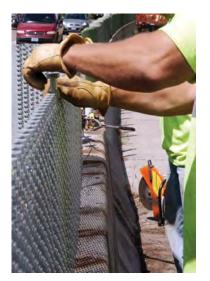
6. Continue to insert <sup>3</sup>/<sub>4</sub>" Post Bolt through the DRC Fabric at the anchor locations. Use the come-a-long to position the bolt over the anchor, keeping the DRC fabric taut.
