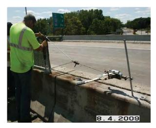
4. Attach the Come-A-Long Cable Assembly to Come-A-Long ratchet provided by installer.
