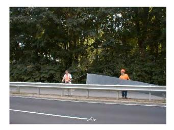
7. When joining two rolls of DRC Fabric, use the splice plates provided. Insert the <sup>3</sup>/<sub>4</sub>" post bolt through the splice plate first and then through the DRC Fabric. Secure the bolt to the two-hole splice angle bracket as described in Step 3. Trim the fabric and leave one row of fabric beyond the post bolt when trimming. Detach the come-a-long from the remaining piece of DRC Fabric.
