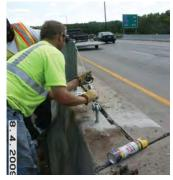
Tighten the <sup>3</sup>/<sub>4</sub>" turnbuckle finger tight. See attached detail drawing.
