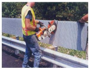
8. Secure the bolt in the anchor and trim the fabric. Leave one row of fabric beyond the post bolt when trimming. Detach the come-a-long from the remaining piece of DRC Fabric. Next insert the second <sup>3</sup>/<sub>4</sub>" post bolt through the same splice plate and then through the "new" roll of DRC Fabric in the first row beyond the starter tab. Re-attach the come-a-long to DRC Fabric.
