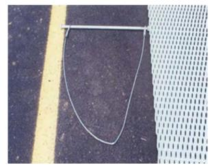
3. Attach the Come-A-Long Cable Assembly provided by Transpo to the opposite end of the DRC Fabric using the <sup>3</sup>/<sub>4</sub>" steel post provided. Please note: Do not use Post Bolt.
