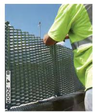
Next insert the second <sup>3</sup>/<sub>4</sub>" post bolt through the same splice plate and then through the "new" roll of DRC Fabric in the first row beyond the starter tab. Attach the post bolt to the angle bracket as shown, using a nut above and below the angle bracket. Re-attach the come-a-long to the opposite end of the DRC Fabric.
