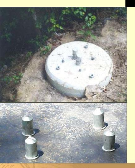
Couplings and hardware are hot-dip galvanized in accordance with ASTM A153.
